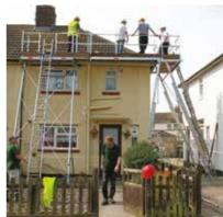
Two or more Easi-Dec platforms can be securely linked with our Catwalk to provide a continuous fully guarded platform compliant with edge protection requirements set out in EN13374.
