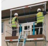
Window-Dec is a purpose designed platform which incorporates a lifting mechanism for window replacement. The fully protected work platform has an opening in the base to allow windows to be lifted through, safely and securely.
