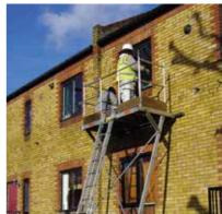
The original Easi-Dec platform provides safe, rapid access to roofline level, whilst spanning building obstructions such as porches and windows.
