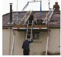
Solar Platform has been specifically designed to allow safe access up to roof level for solar installation, repair and maintenance. The Solar Platform is a 2m wide platform on adjustable legs with a rolling window bar, strap operated legs and a purpose designed hoist for lifting Solar Panels to roof level.
