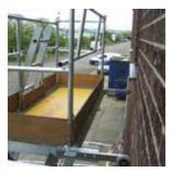
**Stand-Off Kit:** Allows safe access over deep soffits. The kit comprises a pair of 20cm Stand-Off arms which safely position the platform away from the building
