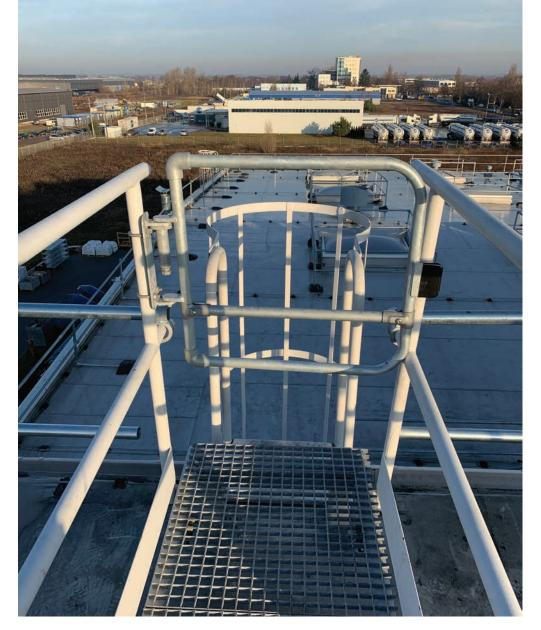
OSHA has also recently determined that chains do not provide suitable protection for ladderways or hatches as they rely on the user putting them back in place once they've accessed the roof.
