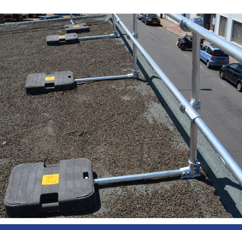
This overview details the introduction of BS13700:2021 and latest guidance for the Recertification of Permanent Counterweighted Guardrail Systems (PCGS), from the perspective of the Duty Holder (normally the Building Occupier).
