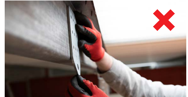
Fig. 1: Incorrect - bracket bends towards you
